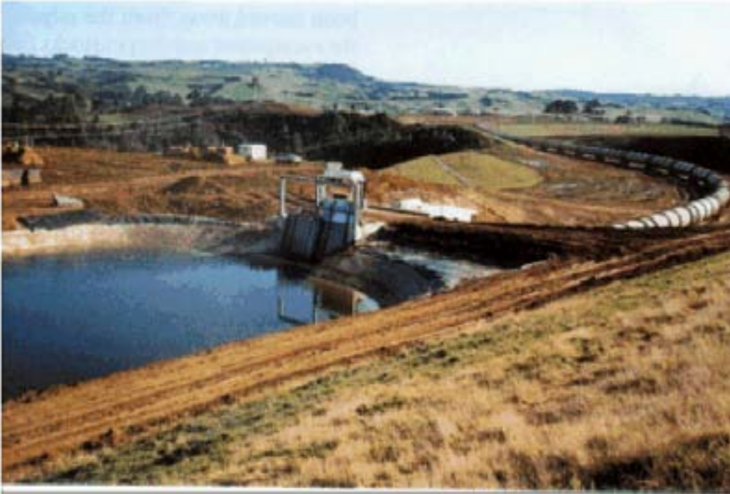
Photo 4-9 Ruahihi canal solution
