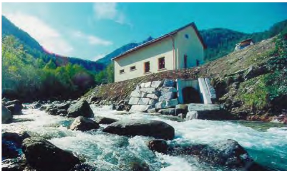
Photo 6.1: Overview of a typical powerhouse
