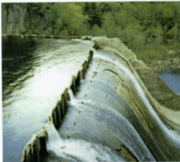
Figure 5.10: Flashboards, articulated & embedded
