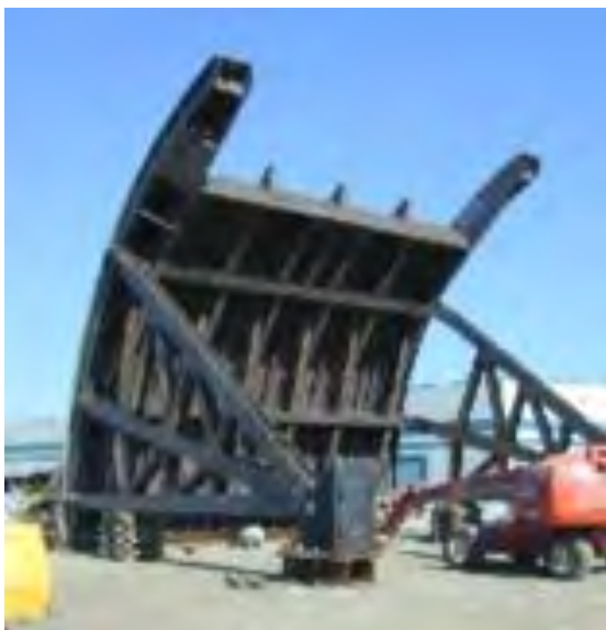
Photo 5.15: Tainter gate (left) and housing of its sector on a concrete pier
