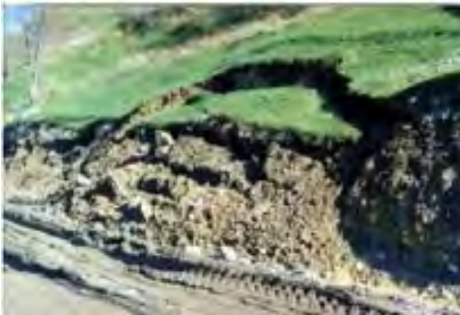
Photo 4-2 Local instabilities generated during the excavation works
