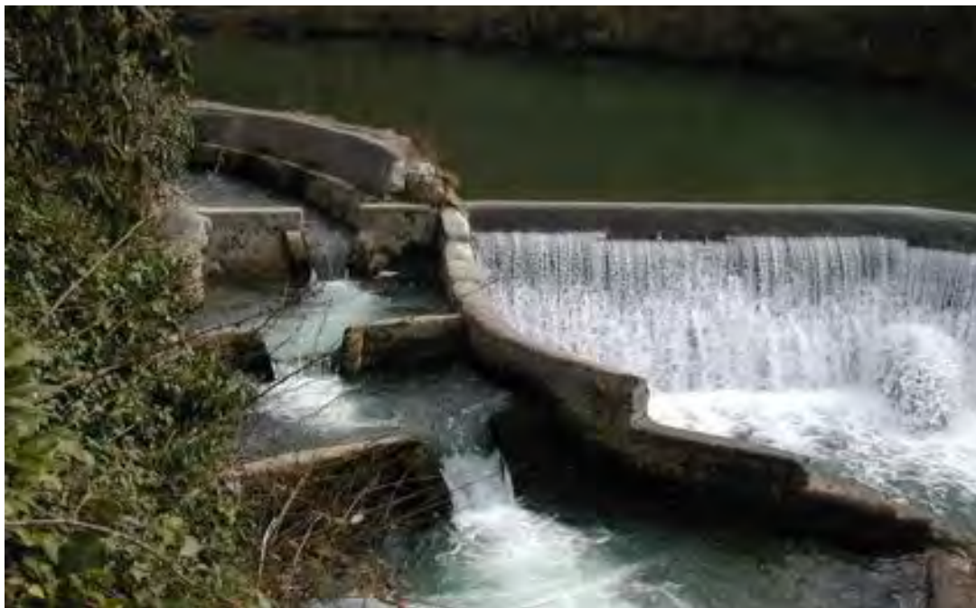
Photo 7.13: Fishpass of rustic construction
