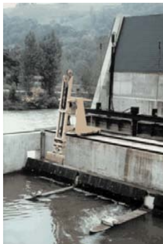
Photo 5.10: Telescopic hydraulic cylinders
