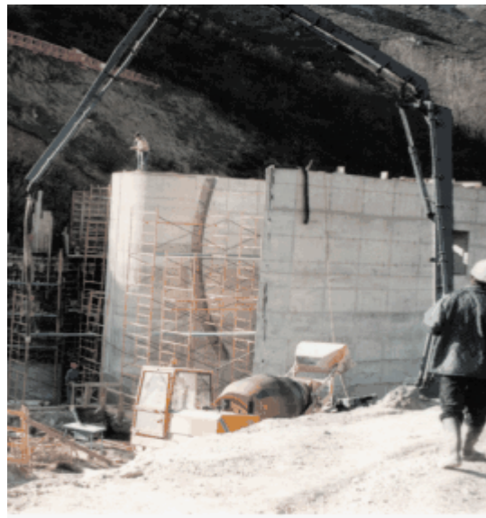
Photo 5.15: Tainter gate (left) and housing of its sector on a concrete pier
