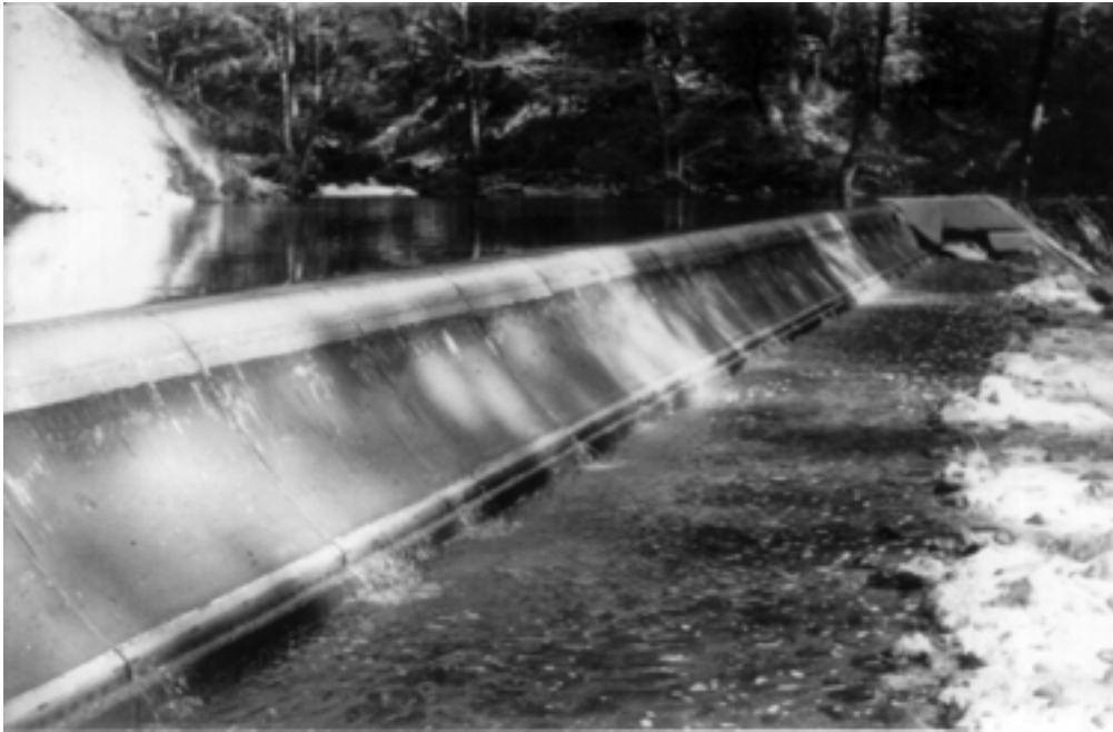
Photo 7.17: Coanda Screen in situation
