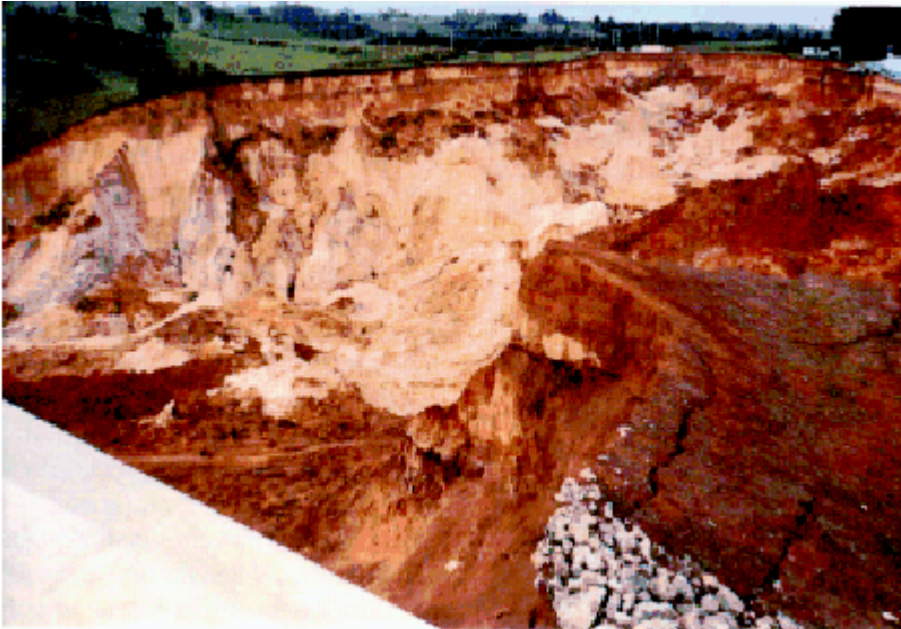
Photo 4-8 The effects of failure
