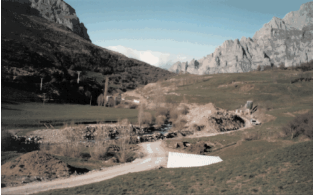
Photo 7.5: Construction phase – excavation
