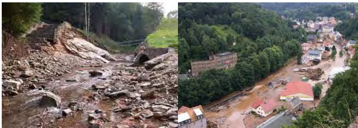
Photo 5.3: Failure of a small dam, the breach and the flooding downstream
