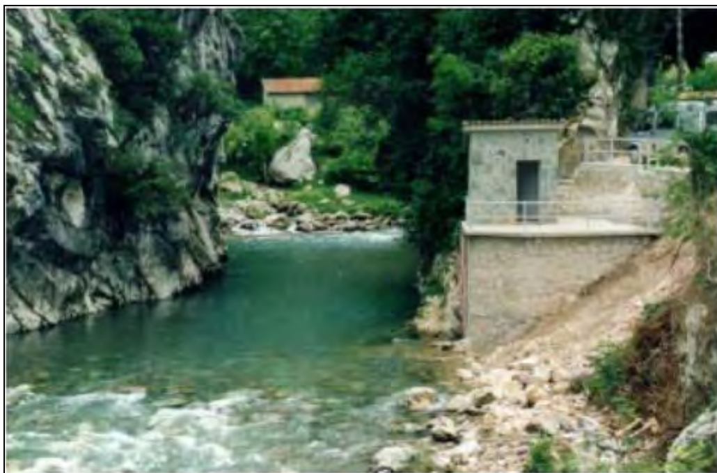
Photo 3-1 Gauging station in a river
