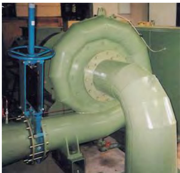
Photo 6.3: Horizontal axis Francis turbine
