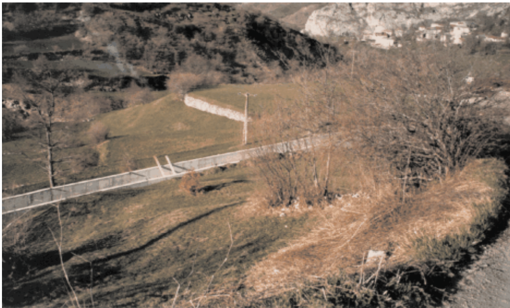
Photo 7.6: Construction phase – concrete canal
