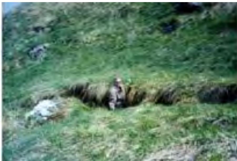
Photo 4-3 One of the existing sliding scarps before the beginning of the works
